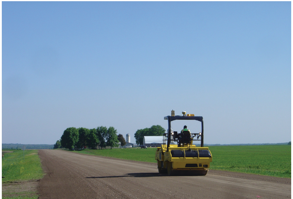
A double drum IC roller pre-mapping the granular base at Route 4, MN under the TPF-FHWA IC study.
