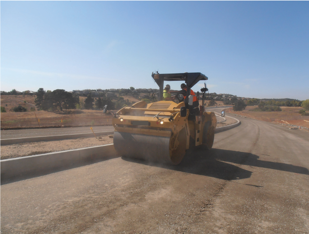
A double drum IC roller conducting pre-mapping under the FHWA-TXDOT IC Retrofit study.
