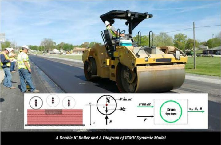
*A Double IC Roller and A Diagram of ICMV Dynamic Model*
