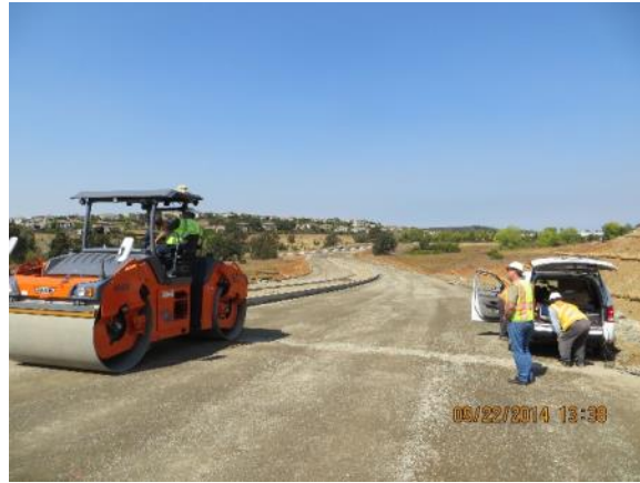
Figure A.5.6. Data collection during stationary vibration
