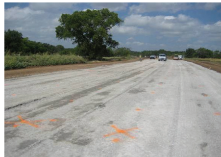
A day after compaction on flex base
