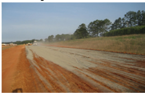
Placement of cement on moist-conditioned subgrade
