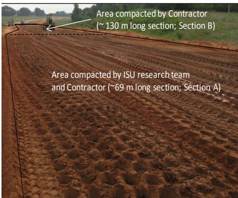
5.5% cement treated granular base
