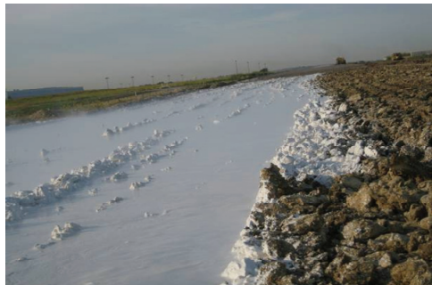
Ponding of lime slurry on the scarified subgrade
