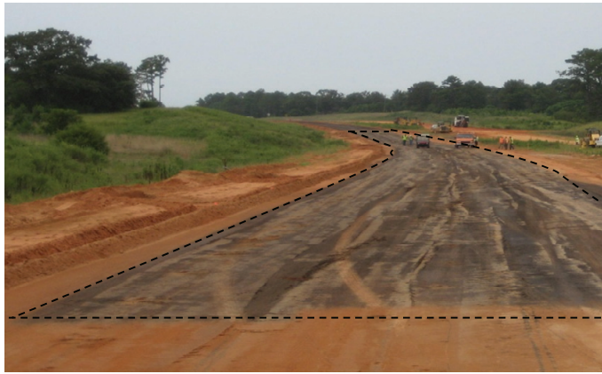
5-day cured 150mm thick cement treated granular base
