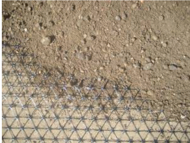
Figure 74. Photographs of TB4 during placement of TX5 geogrid and salvage base layers
