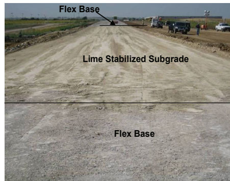
Flex base and lime stabilized subgrade
