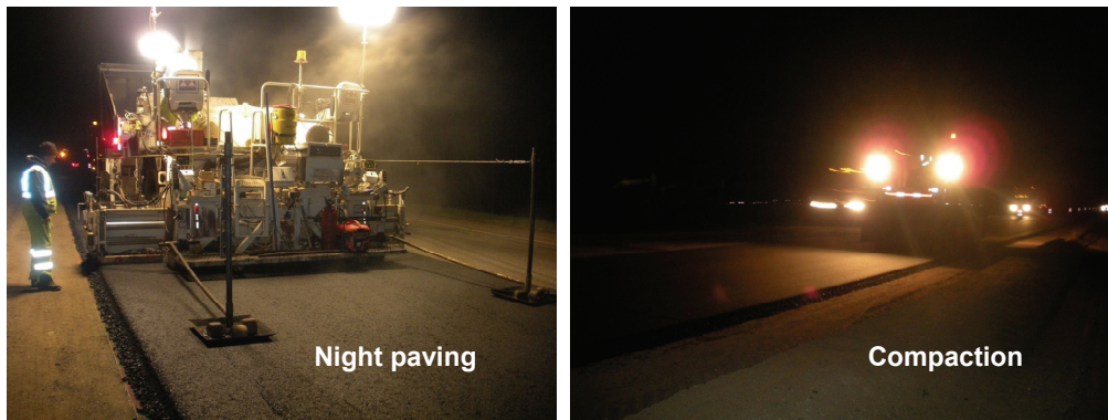
Figure 145. Night paving and HMA compaction.
