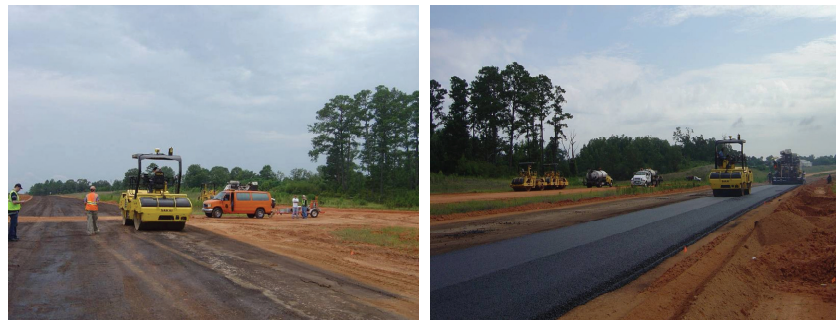
Figure 106. Mississippi HMA IC demonstration.
