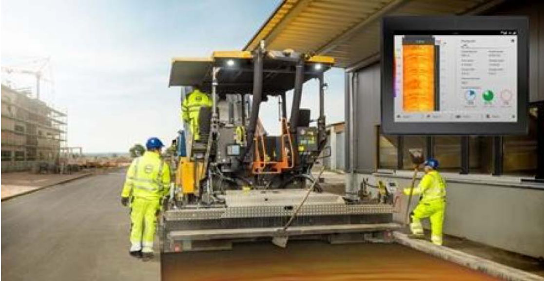
Figure 5. Volvo PaveAssist thermal imaging system
