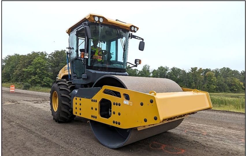
Figure 1. Single-drum roller used in this study. (Source: The Transtec Group, 2023)
